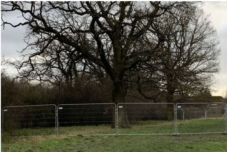
Figures 3 & 4: Examples of tree protection measures
