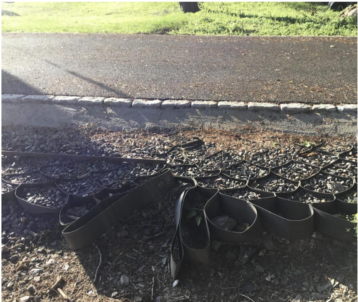
Figure 8: Example of permanent tarmac using Geocell or similar. Exposed Geocell is only there to show that it is present but would normally be covered/under the road.
