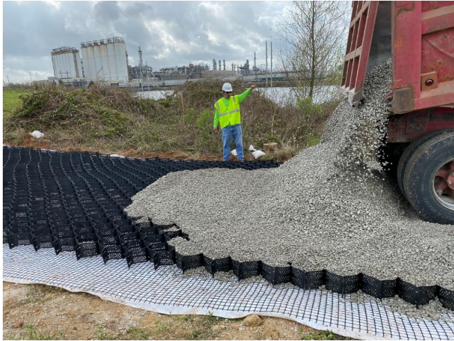
Figures 6 and 7: Examples of ground protection for heavier vehicles: Geocell technology (available in India)
